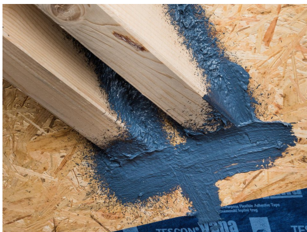
9. The finished joint at a double collar tie penetration
