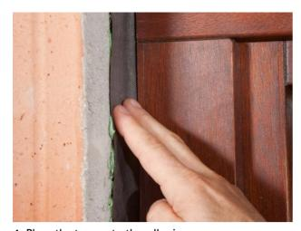
4. Place the tape onto the adhesive
