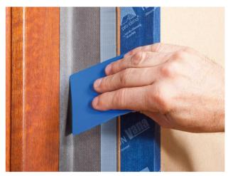
5. Press firmly to secure the CONTEGA EXO in place
