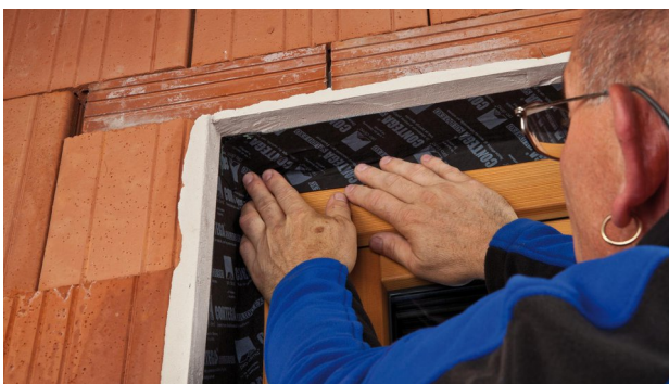
7. Stick the corners and around the circumference of the window Continue sticking the entire window (frame and soffit) in the same manner. Ensure that the corners are stuck over.
