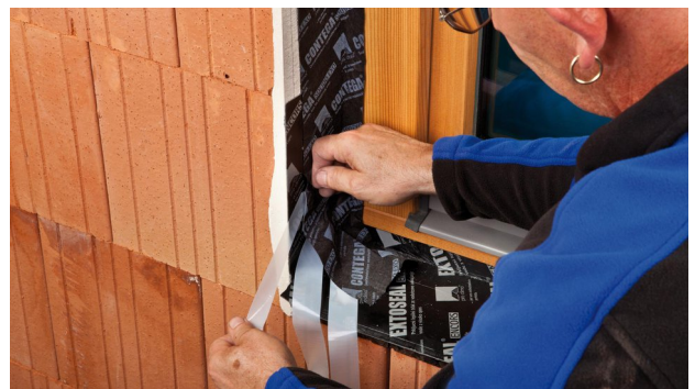
6. Stick to the soffit allowing for slack Remove the backing paper strip and gradually stick the tape in place on the soffit. Leave slack for expansion so as to allow for relative motion between components. Stick the tape to the window sill.
