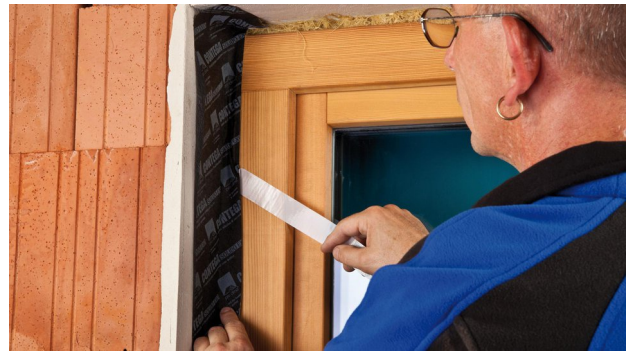
4. Stick to the frame Remove the narrow backing paper strip. Put the CONTEGA SOLIDO EXO in place using the full width of the adhesive strip and allowing for an excess of 2 cm beyond the corner of the frame. Stick the excess tape to the adjacent soffit side.
