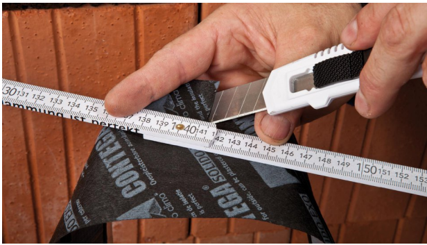
3. Cut the window sealing tape CONTEGA SOLIDO EXO Add approx. 4 cm to the height of the frame and cut this length of tape.
