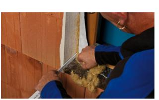
**5. Installing the window and insulating the joint** Fold in the CONTEGA SOLIDO SL-D and install the window professionally. Use a suitable fastening system.
