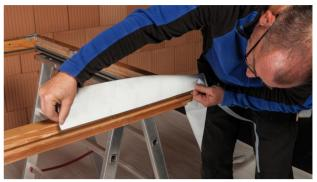
**2. Sticking to the side of the frame** Remove the single release film strip on the printed side, position it on the side of the frame and then gradually stick in place. The printed side of the tape must be facing the window (upwards) here. Rub tape firmly into place using the pro clima PRESSFIX.
