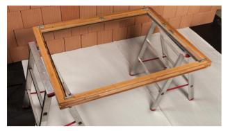
**1. Masonry or timber structure** CONTEGA SOLIDO SL-D is fitted before the window is installed. The frame is laid out flat. The interior side is facing up.
