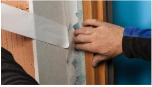
**5. Sticking to the soffit, allowing for slack** Remove the second (wide) release film strip and gradually stick the tape inplace on the soffit.
