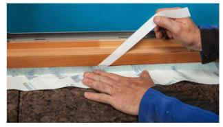
**6.** Sticking the tape to the circumference of the window Continue sticking the rest of the window (frame and soffit) in the same manner.
