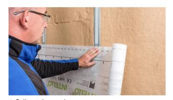
**4. Roll out the membrane**... and press it onto the adhesive tape.
