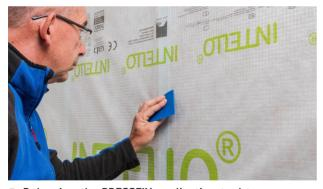
5. Rub using the PRESSFIX application tool to secure.
