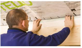
11b. Sealing to roughly sawn timber
