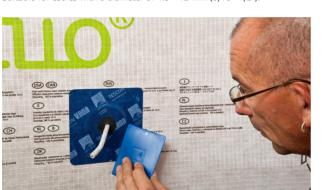
**3. Stick the grommet and rub it firmly in place** Stick the grommet to the subsurface and rub it firmly in place. Ensure that there is sufficient resistance pressure.
