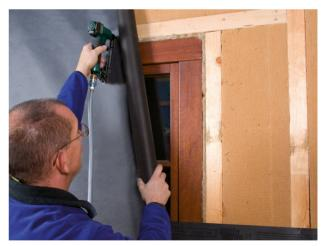
**8a. Sticking to windows** Install membranes continuously over window openings and attach them all around the window using a stapler. Then cut open the opening using a utility knife.
