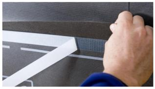
**4. Taping over the overlaps** Gradually remove the release film from DUPLEX and stick the overlapping membrane, ensuring that there are no folds or tension.
