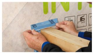
**5. Bonding with the short independent adhesive strip** A tape with a 12/38 mm split is ideal for bonding to components that will subsequently by covered only by a thin layer, e.g. by plasterboard.
