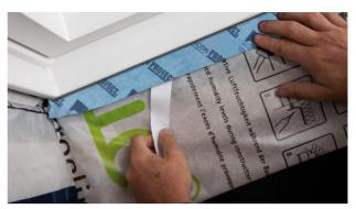
**2. Stick the second independent adhesive strip** Then remove the release film and gradually stick the tape to the second surface (in this case, the soffit).
