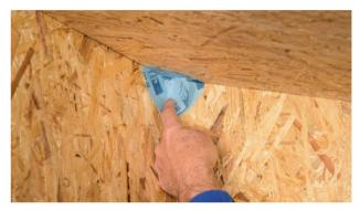
**4. Rubbing the patch firmly into place** This step can be carried out in a manner that is kinder to your hands by using the pro clima PRESSFIX application tool.
