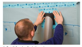
**6. Detail for pipe feed-through** Pull the pro clima ROFLEX pipe grommet over the pipe and stick it to the airtight surface in an airtight manner using UNI TAPE.
