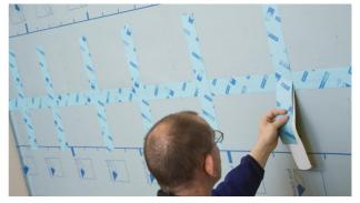
**9b. Detail for blown-in insulation material** Alternatively: under certain conditions, the installation of relief strips at maximum intervals of 30 cm (12") may be sufficient. It is your responsibility to verify this on site.
