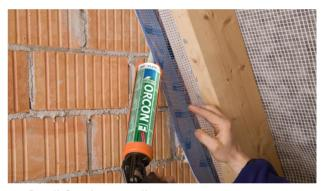
**4a. Detail for plaster sealing tape** Defined plaster sealing using pro clima CONTEGA PV. Attach fleece to the masonry at discrete points using ORCON F or ORCON CLASSIC. Please note: there must not be any hollows under the tape.
